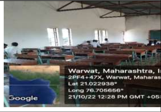
Class Rooms (Old Buildings)
