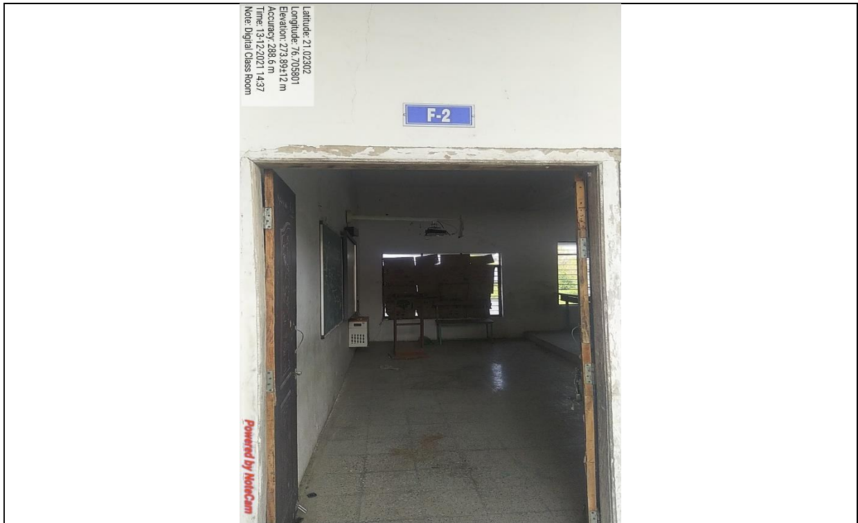
Photo 7: Calsroom with ICT Facility available ( Smart Board and LCD Projector)
