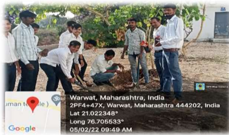
Making ditch for watering plants 5 th February, 2022
